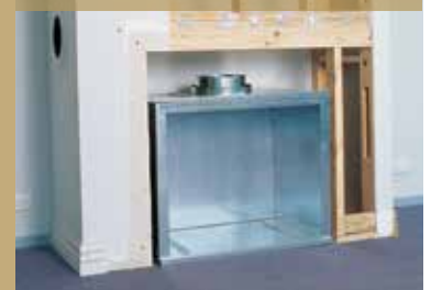
Zero Clearance Box positioned in framework on 12mm sheet
