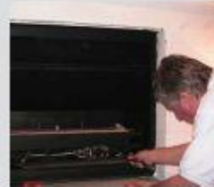
Burner inserted and connected to fixed gas line.
