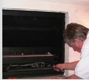
Burner inserted and connected to fixed gas line.
