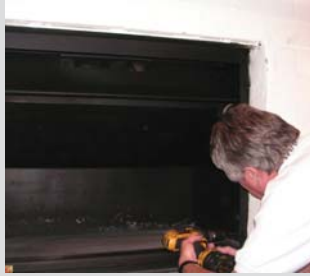
Logpan removed and a 25mm hole is drilled on the RHS of the firebox.
